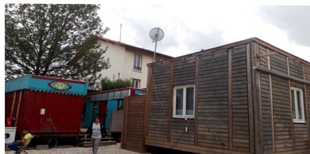
Site of Villensemble project, in Ivry-sur-Seine
