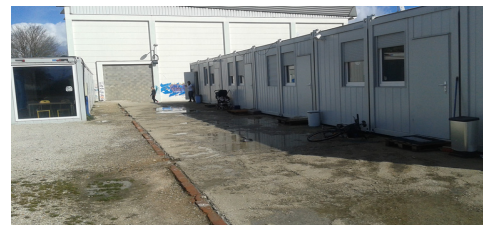
The stabilization village in Dijon
